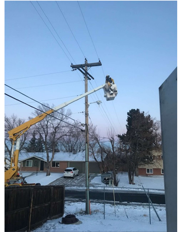
4:52pm Reconnecting Power to the Pump House
