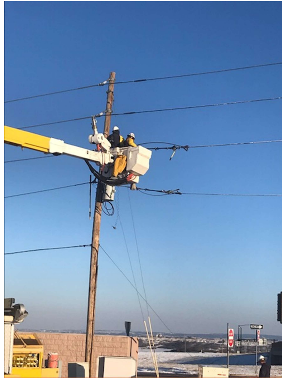
3:43pm Finishing the Last Two Splices
